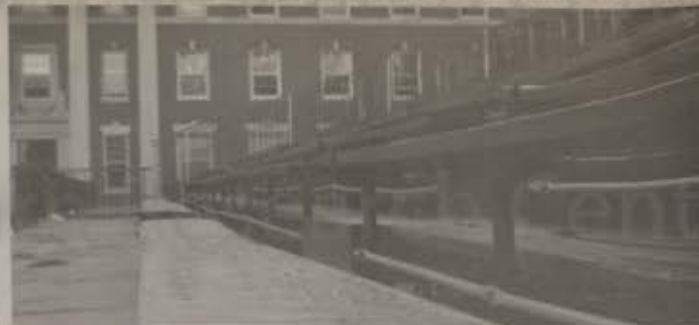
In preparation for graduation, students are forced to find routes through bleachers and construction workers that are building the bleachers on the Yard to get to class.
