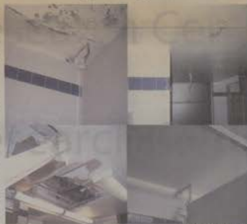
(Top/Bottom Left) Restrooms before repairs took place over Spring Break. (Top/Bottom Right) After repairs.
