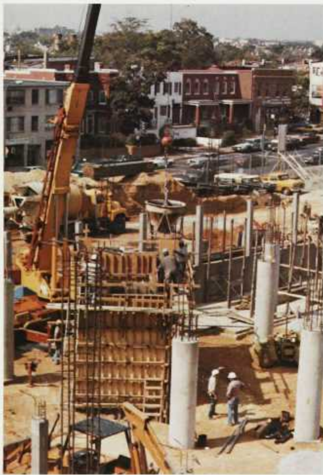
The laying of the foundation of the new School of Business.
