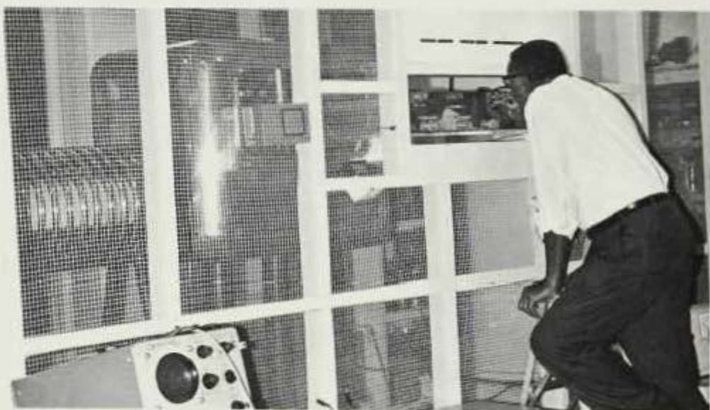
Dr. Ferguson makes adjustments on proton accelerator used in a project on Cancer Research.
