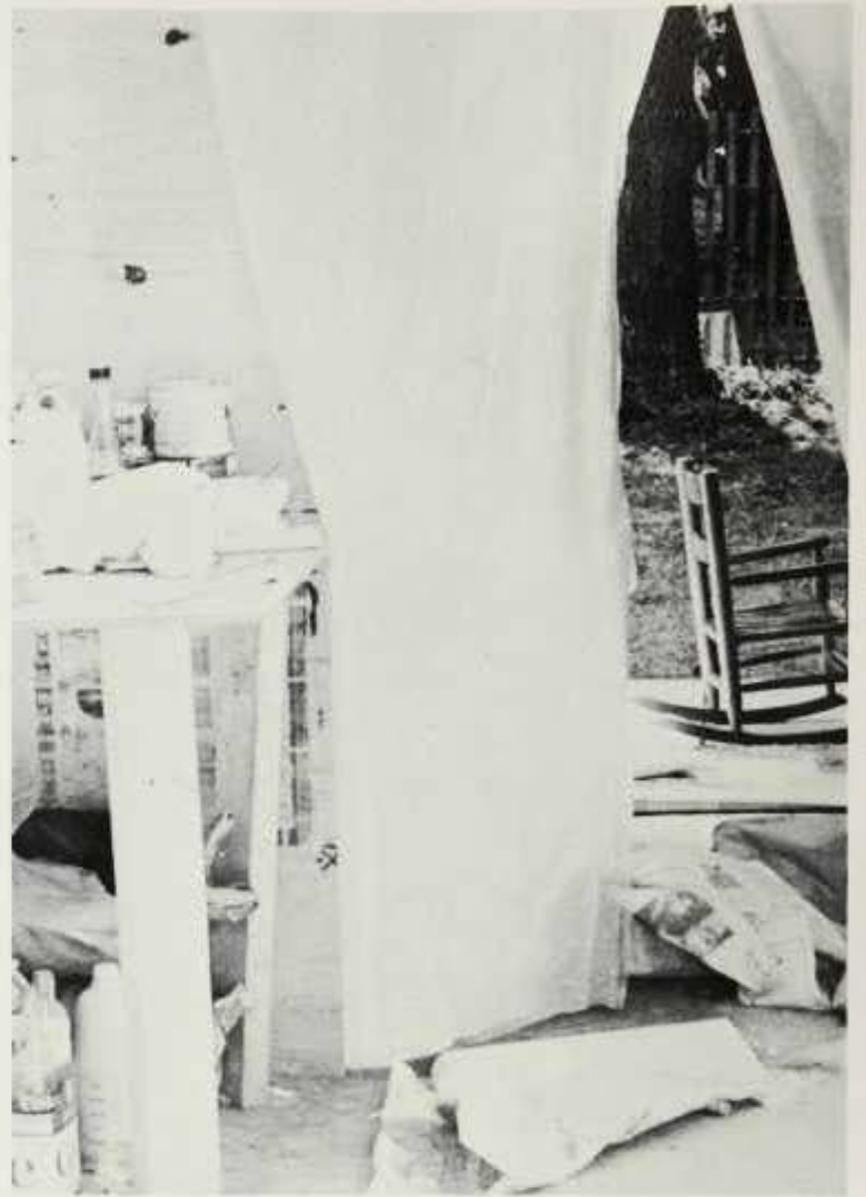
Conditions inside and outside of the wooden huts were terrible
