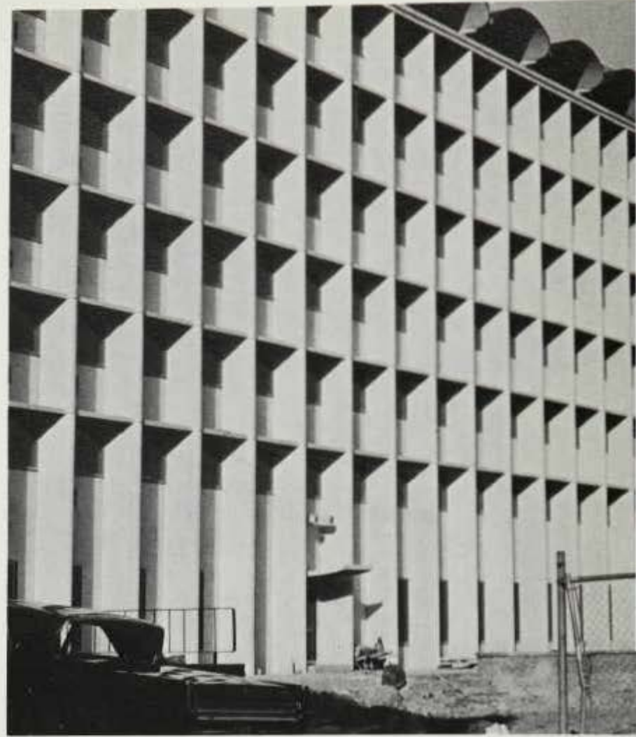
The new women's dorm nears completion for the fall semester.
