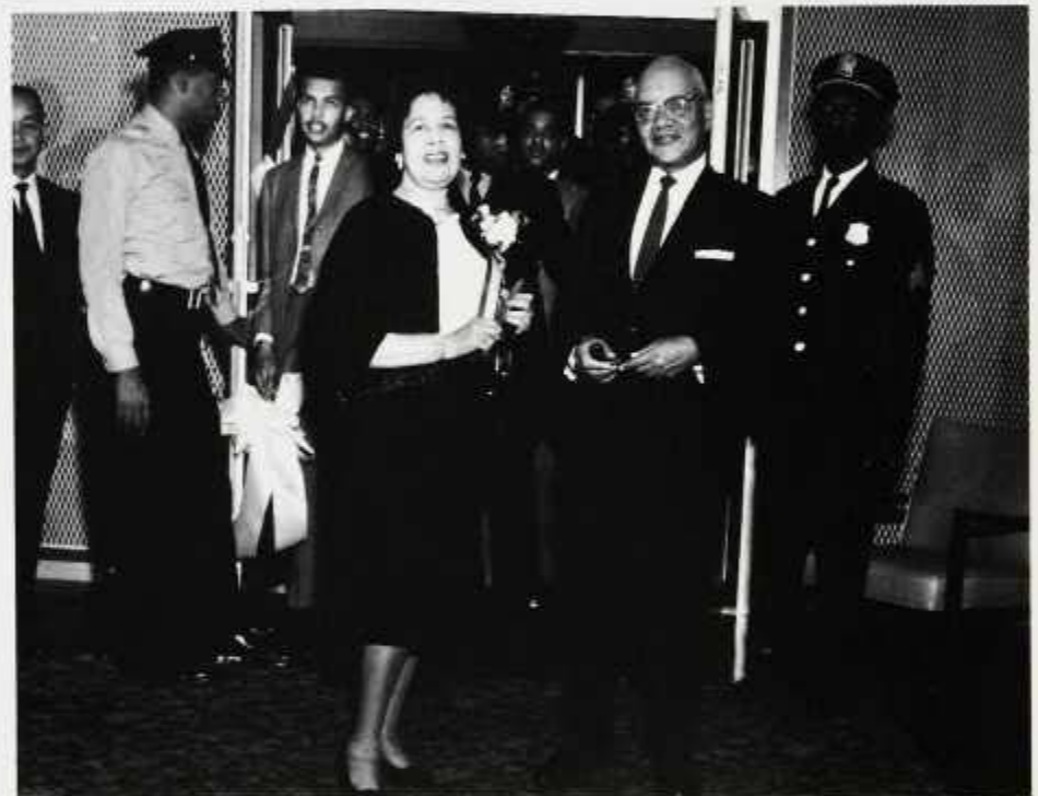
A pose for the photographer before touring the remodeled building.
