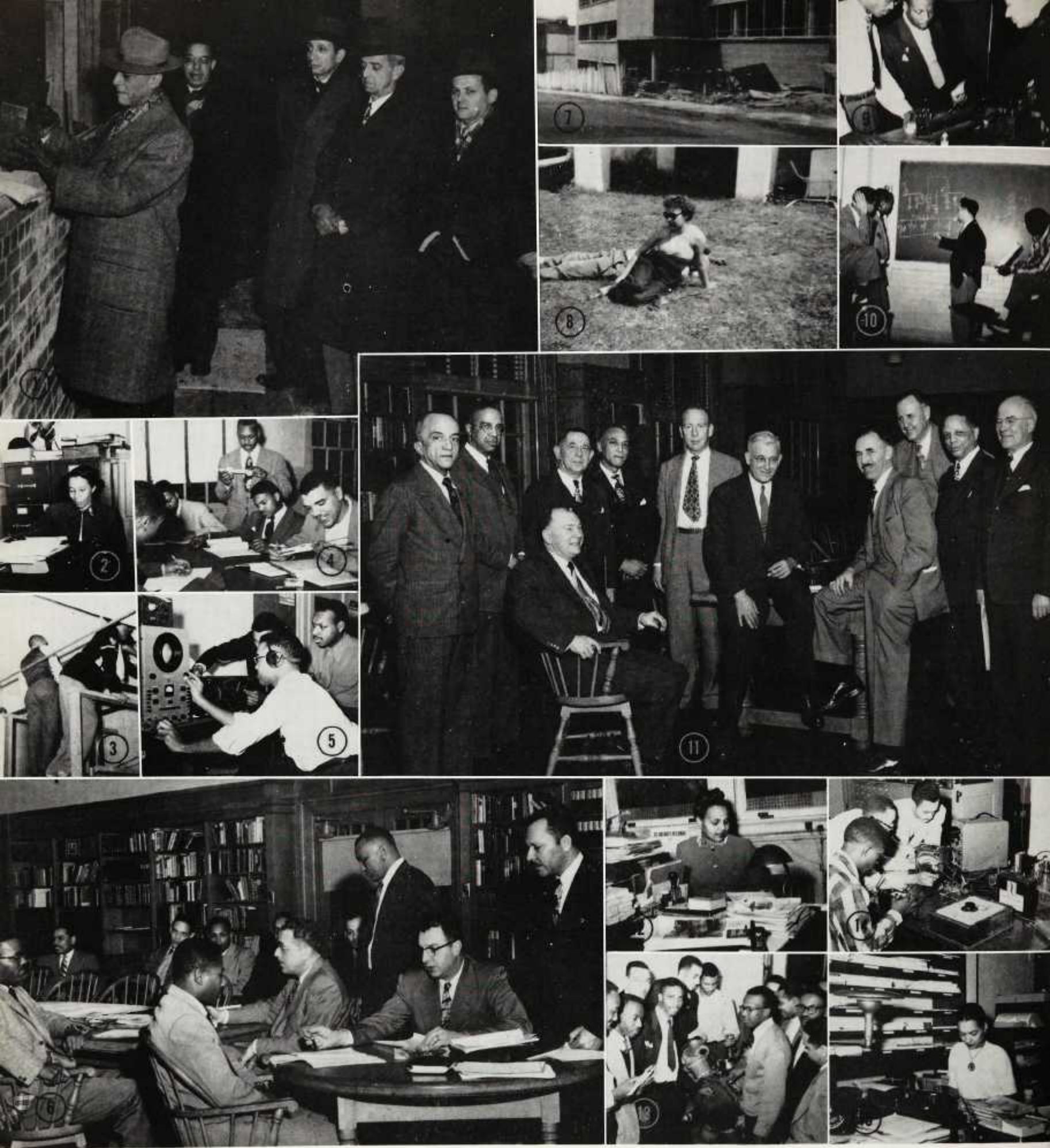
1. Dedication services for the new E. & A. Building. 2. Mechanical Engineering office. 3. Hydraulic lab. 4. Problem session. 5. Howard Amateur Radio Group at work. 6. T. V. A. interviewers. 7. Progress on the new E. & A. Building. 8. E. & A. picnic. 9. Experimenting with D. C. Circuit and machinery. 10. Instructions on Electronics. 11. American Society of Engineering Education. 12. Dean Downing's outer office. 13. Instruction on Internal Combustion engines. 14. Experimenting in Communications. 15. E. & A. Library Receptionist.
