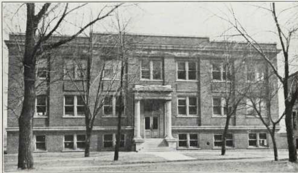
APPLIED SCIENCE BUILDING
