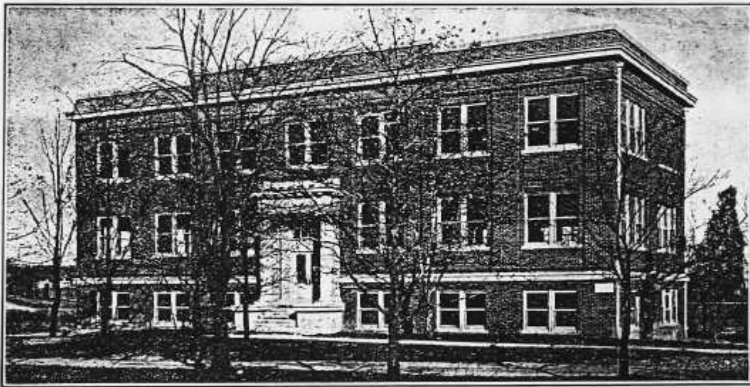
HALL OF APPLIED SCIENCES AND INDUSTRIAL ARTS
