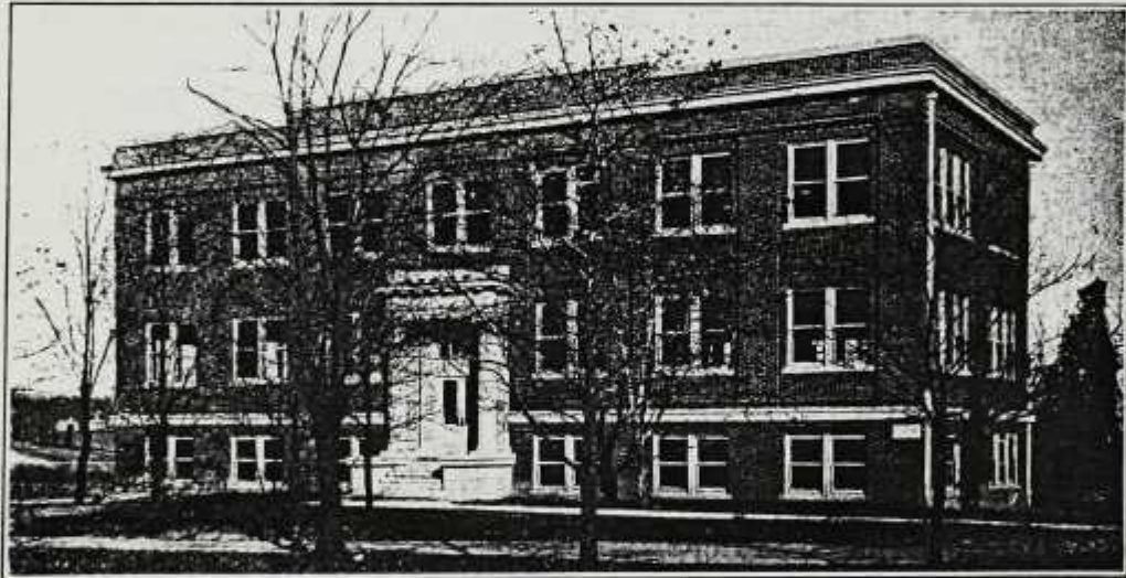
HALL OF APPLIED SCIENCES AND INDUSTRIAL ARTS.
