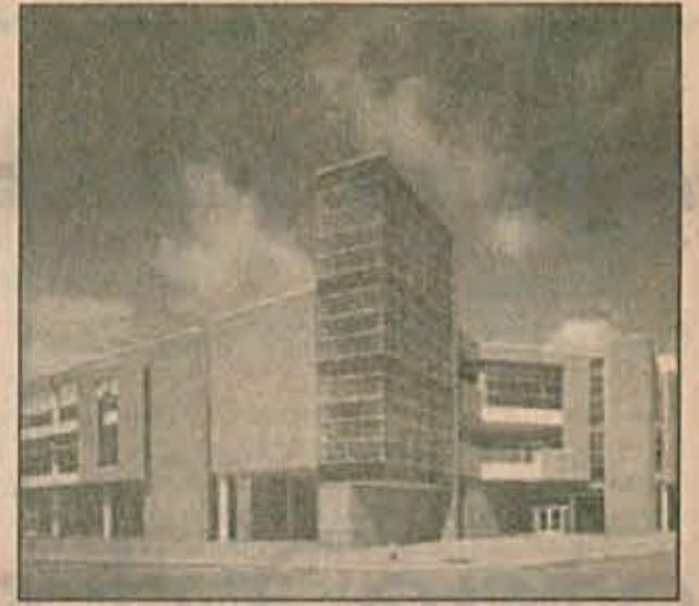
A new dormitory finished at Hampton University
