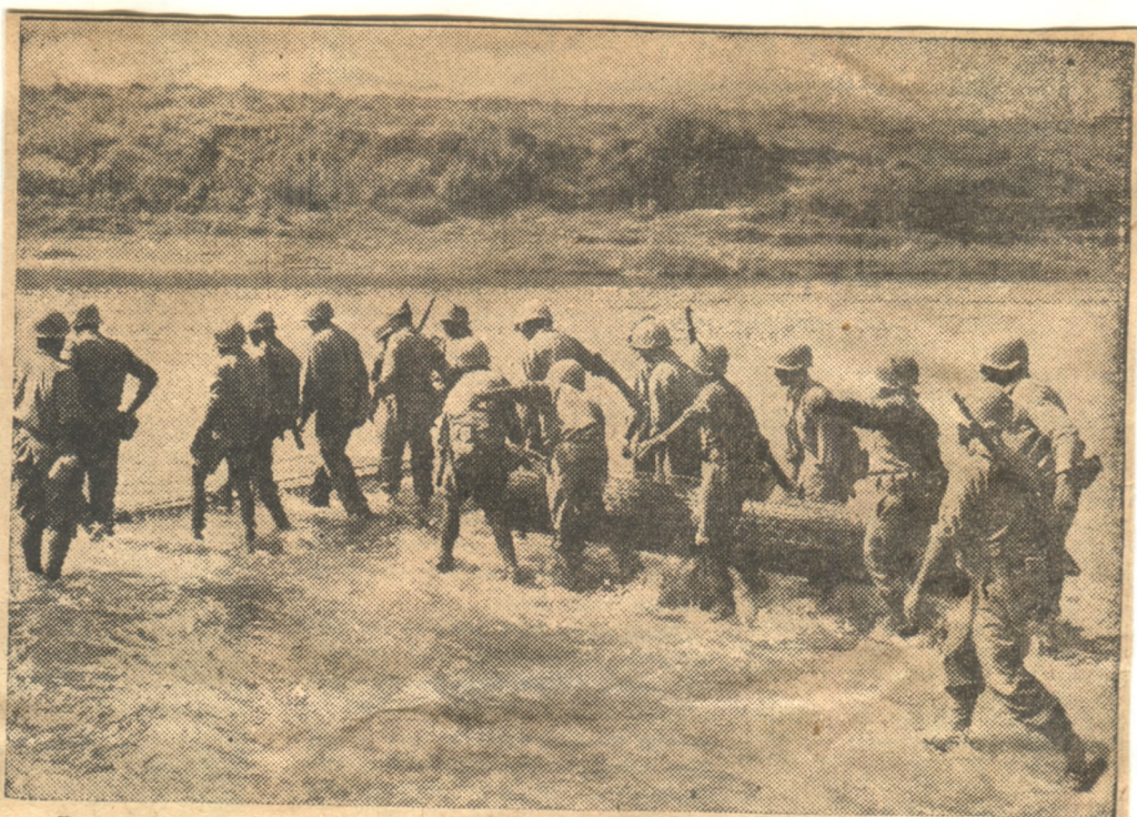
Preparing the Arno River for traffic, these engineers laying down wire netting across which men will walk through the shallow stream. All carry guns for emergency use.
