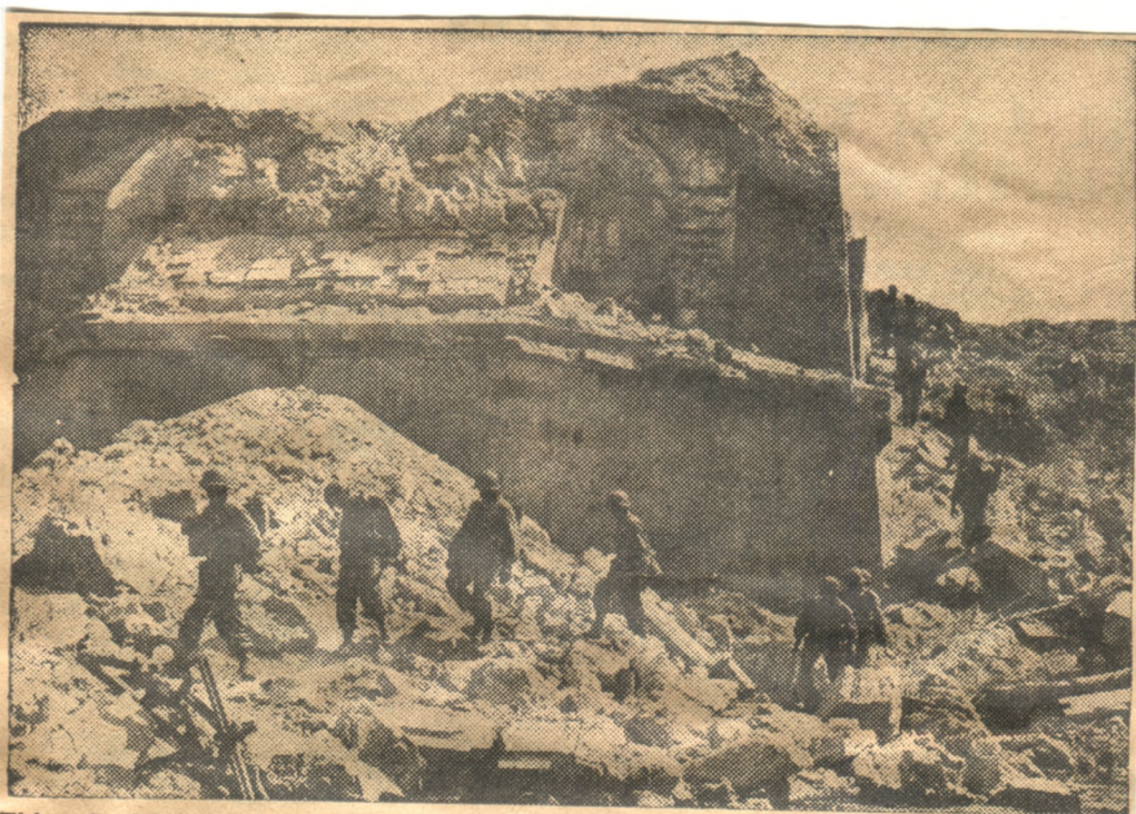
This ruined bridge in the Pontederra area once spanned the Arno River but this is all that's left as units of the 92nd Division push through toward German positions on the vaunted Gothic line.
