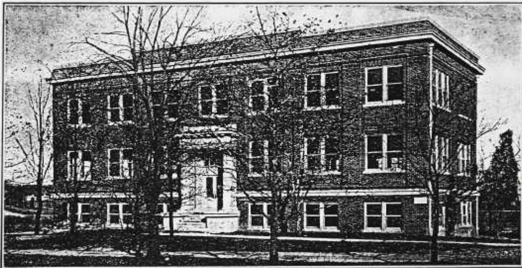
HALL OF APPLIED SCIENCES AND INDUSTRIAL ARTS
